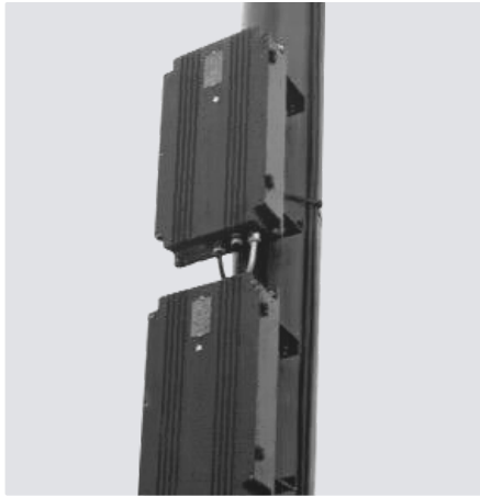
Control Gear fixed on the pole
