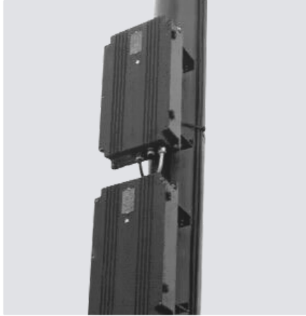
Control Gear fixed on the pole
