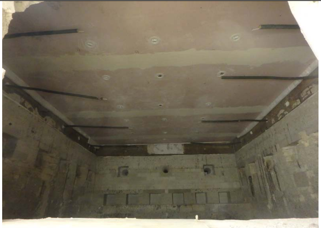
The exposed face of the assembly prior to the start of the test
